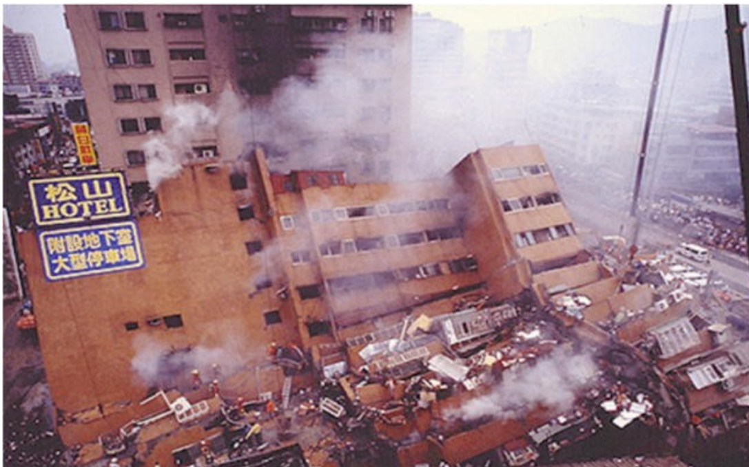
Figure 6. The Dongshing Building collapsed during the 1999 Jiji (921) earthquake (Hsu, 2022).
