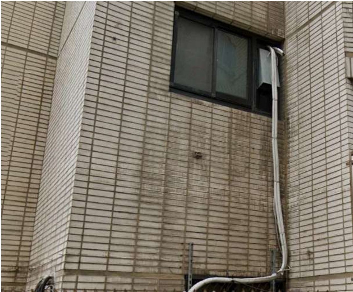
Figure 16. Cracking, spalling, and uneven coloration of Building B's exterior wall tiles (Google Earth, 2022).
