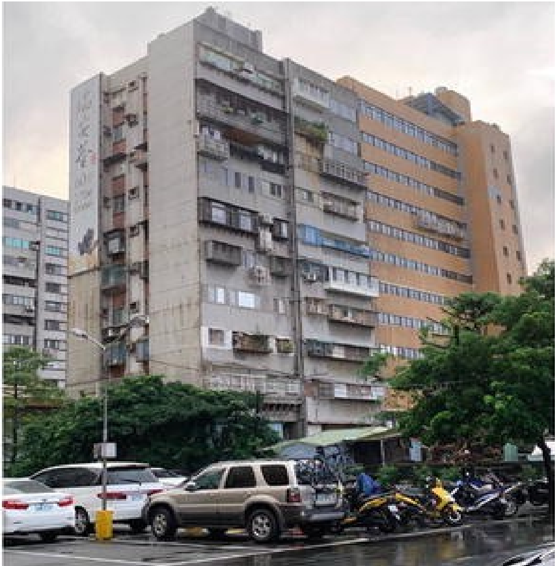
(a) Failure of tilting and subsidence.
