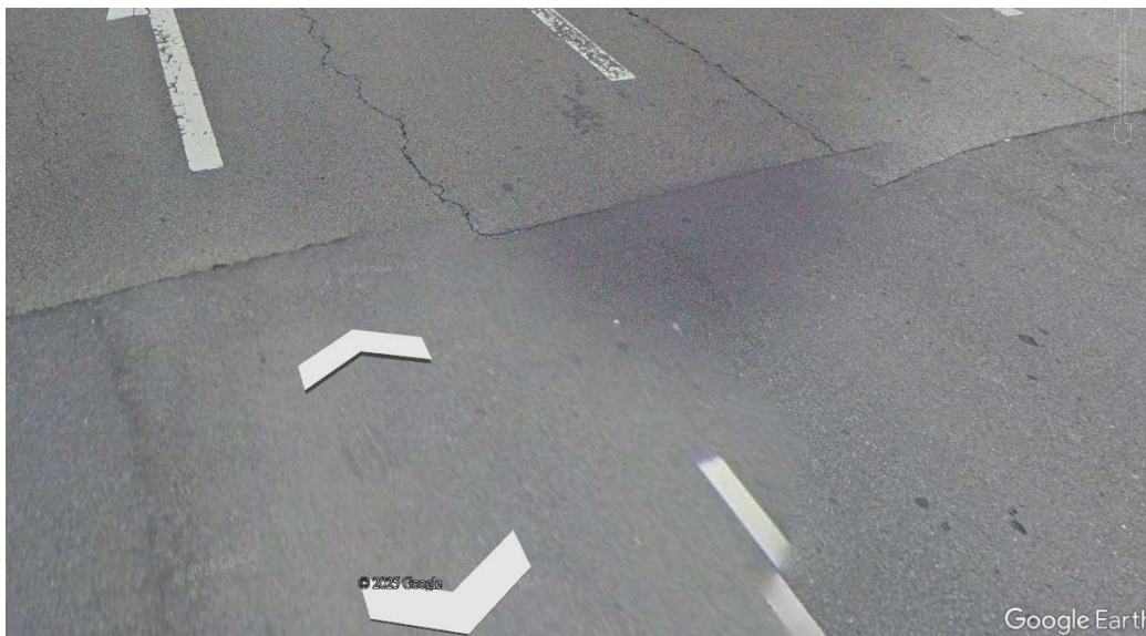
Figure 18. Uneven settlement of the road adjacent to Building D and cracking of the AC pavement (Google Earth, 2022).
